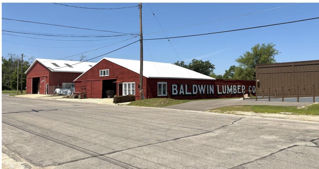
A local lumber, hardware, and building supply business in Baldwin, Lake County, MI (Photo courtesy of Steve Kraft)
